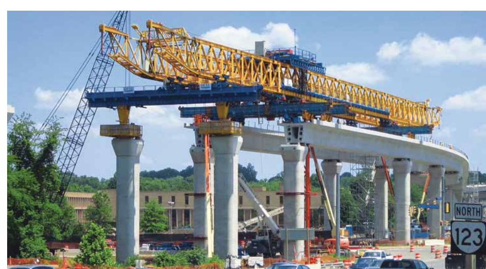
Precast, Span-by-Span Method
