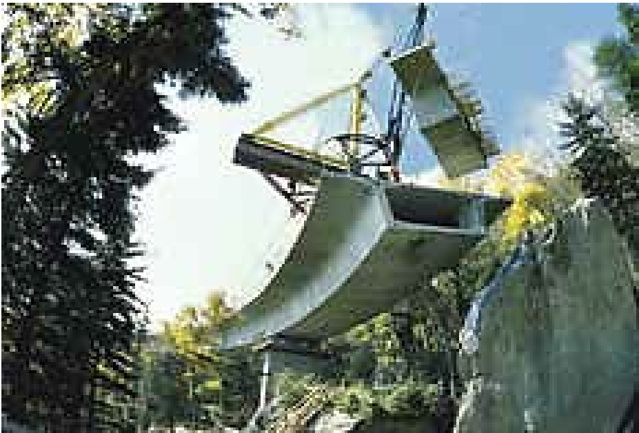
Precast, progressive placement method
