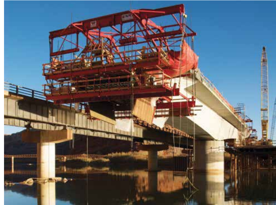
Cast-in-place, balanced cantilever method
