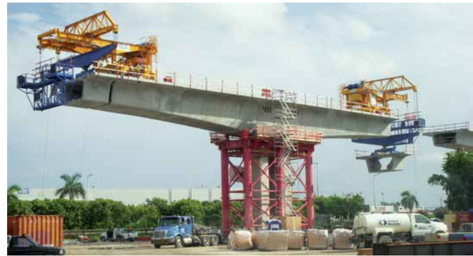
Precast, balanced cantilever method
